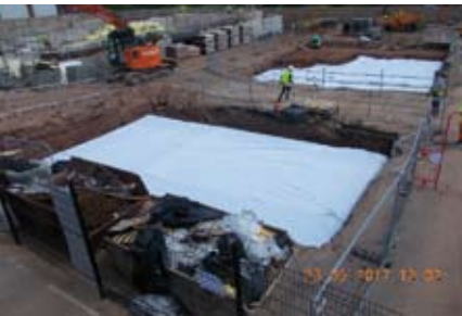
Drainage storage tanks
